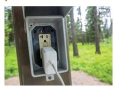
Electrical outlets can be solarpowered and are best located either in a secure place (inside of lockers) or at another central place like the group picnic area.
